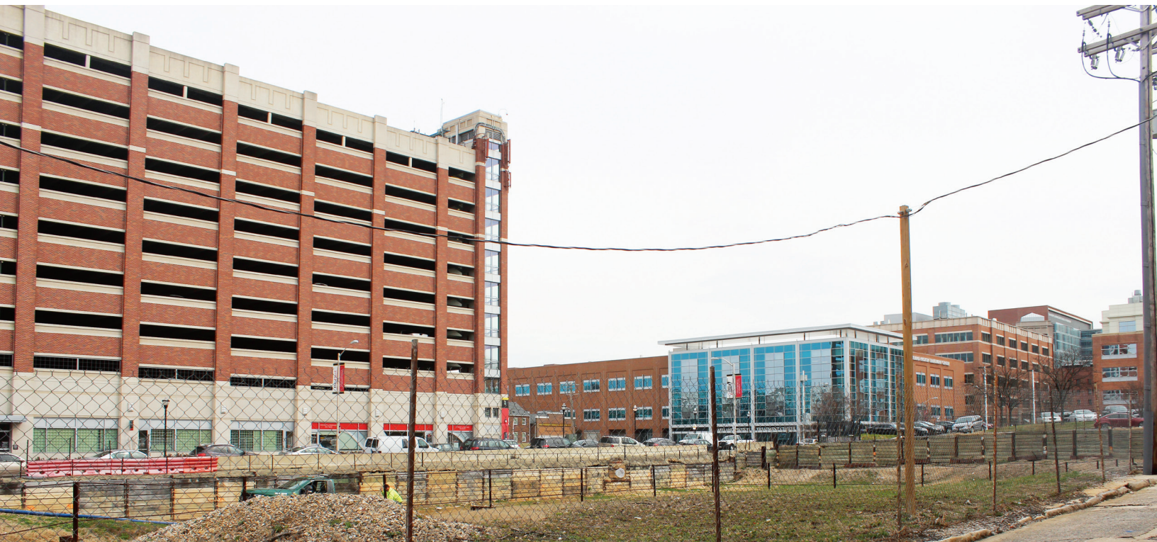
Large construction site in the 800 block of West Baltimore Street.
